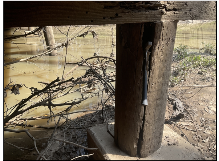
Bent 2 pile 5 is split and hollow at the top
