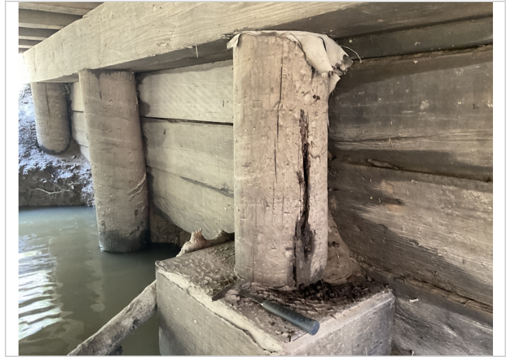
Bent 6 pile 3 has a decayed area 2' long 2" deep
