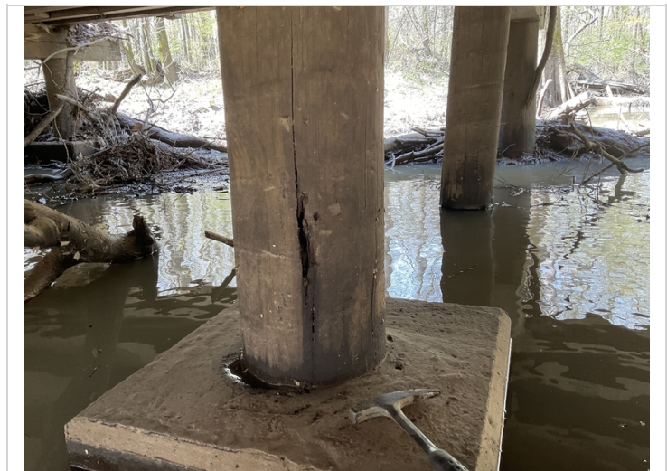
Bent 3 pile 3 split with decay
