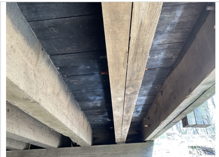
Span 5 girder 12 and 13 replaced with sandwiched beams
