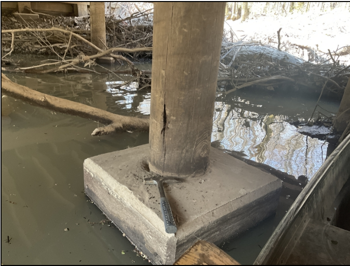
Bent 3 pile 3 is split and decayed.
