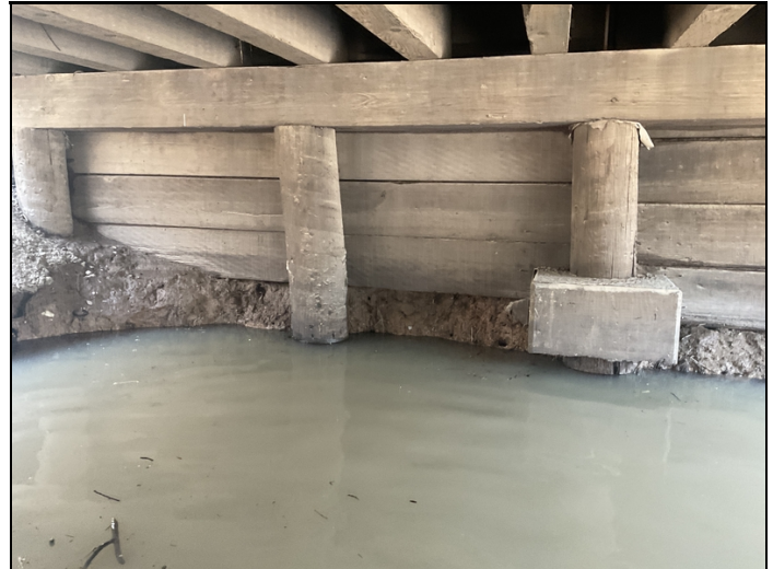
Timber cribbing at bent 6 is being undermined due to channel being block by trees and debris
