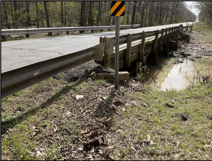
Approach guardrail post laid over due to traffic impact
