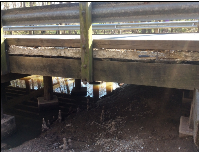
Span 1 left side spalling due to concrete deterioration.
