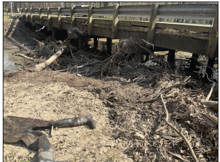
Logs and debris build up on west side of bridge restricting water flow
