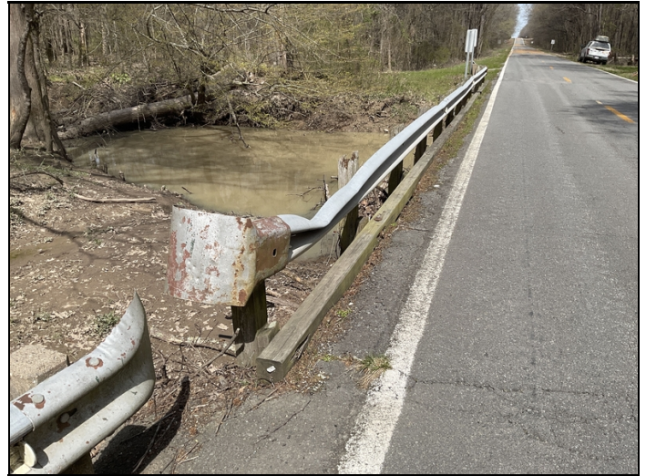
Guardrail damage at southwest end
