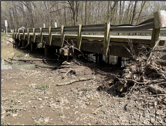
Debris at bent 2 and 3 upstream end
