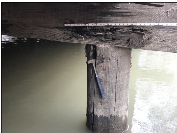
Bent 2 pile 5 is split and hollow at top. 2' of decay on cap.
