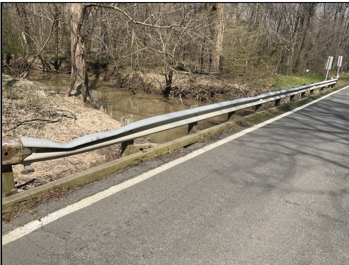
Left bridge rail is damaged
