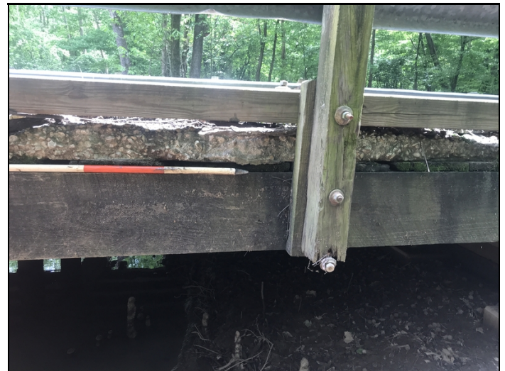
Span 1, left side of concrete deck is spalled
