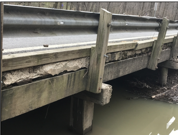
Span 2 and 3 right side of deck has spalls
