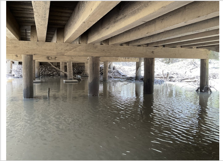
Split at bent 4 pile 3
